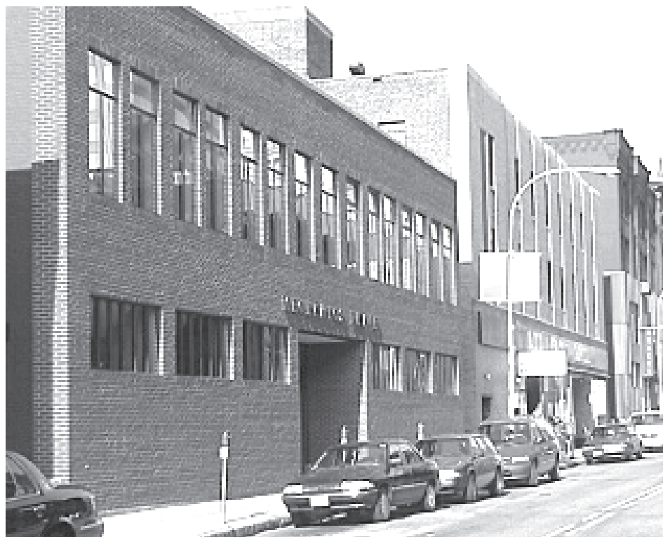
New MCCC Office at 27 Mechanic Street, Mechanics Place, Worcester MA
